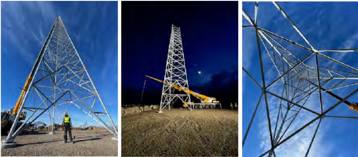
Image 2: The construction of new vertical assets in Lincoln County.
